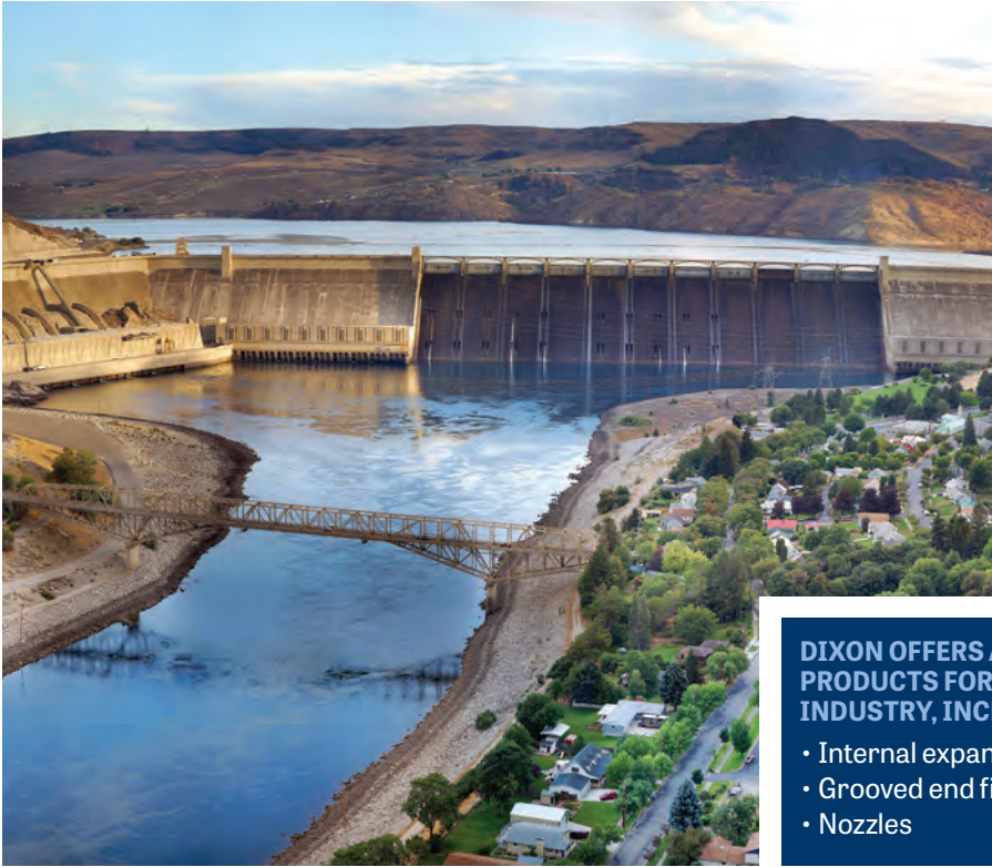
Using the equivalent of Grand Coulee Dam's 12 million cubic yards of concrete, you could build a highway from Seattle to Miami. Photo: Gregg M. Erickson
